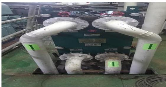
**Gambar 2.78** *Radiator Mesin Propeler*
