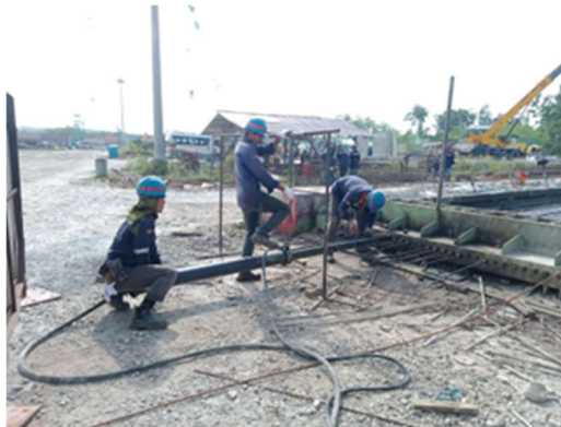
Gambar 3. 6 Proses Initial Strand
