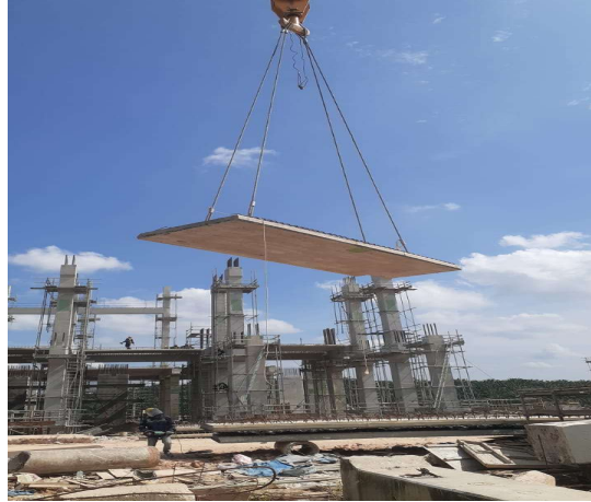
Gambar 3. 23 Proses erection
