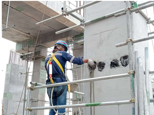
Gambar 3. 29 Proses Grouting
