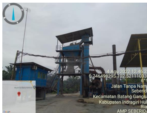
Gambar 2.3 Asphalt Mixing Plant (Sumber : Dokumentasi Lapangan Kerja Praktek 2022)
