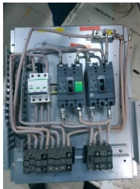
Gambar 2. 22 Rangkaian Power Distributed Panel
