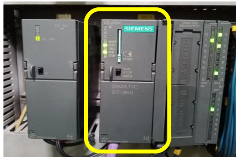
Gambar 3.9 CPU PLC
