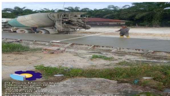
Gambar 3.20 Proses Grufing Rigid
