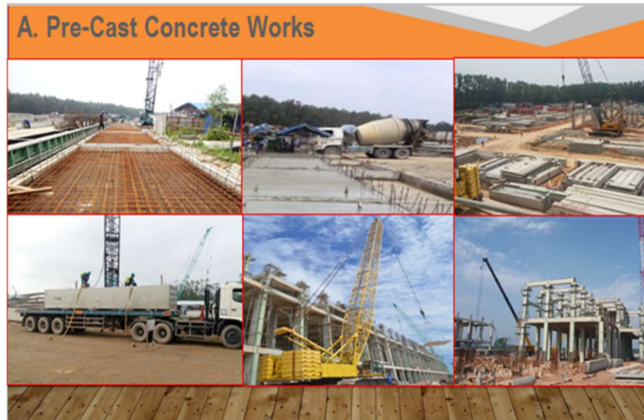
Gambar 1. 5 Pre-Cast Concrete Works
