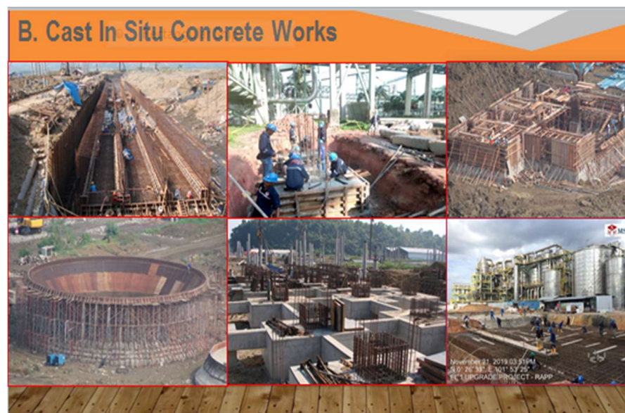
Gambar 1. 6 Cast In Situ Concrete Works
