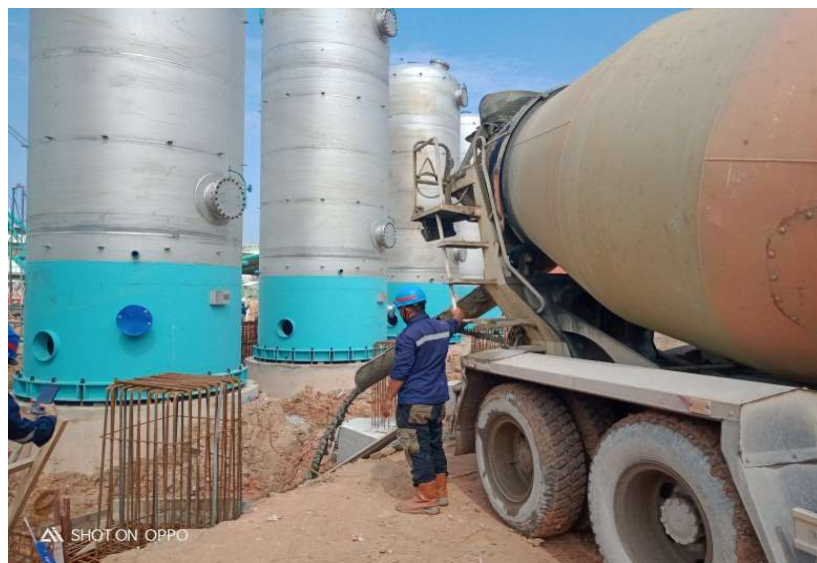
Gambar 2. 12 Beton Ready Mix
