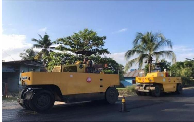
**Gambar 3. 4 Pneumatic Tyre Roller**
