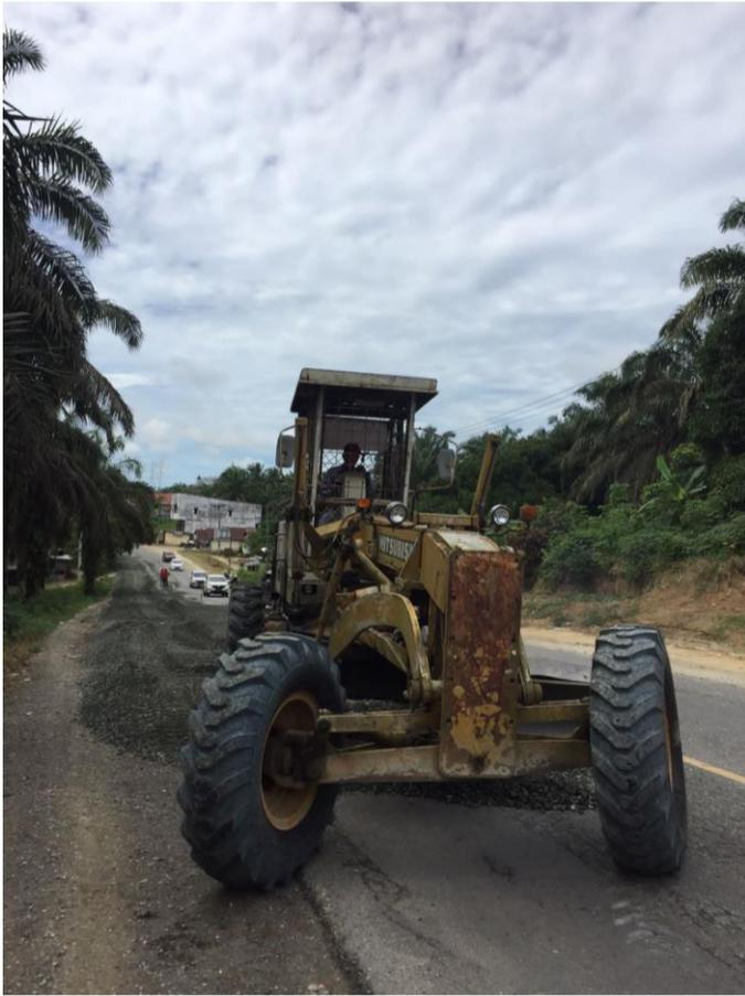
A photograph showing a yellow motor grader with a blade attachment, working on a road shoulder. The machine is positioned on a gravel base, spreading it. The background shows a road with palm trees and a cloudy sky. |            |
