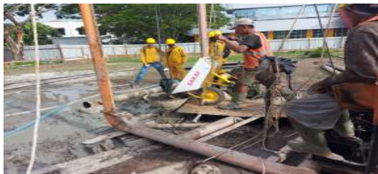
Gambar 3.4 Pengecoran Pondasi Bore Pile
