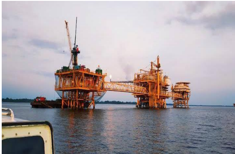
Gambar 1.3 Well Lalang Platform (Sumber : PT.Imbang Tata Alam 2022)
