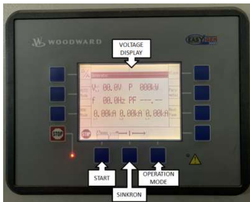
Gambar 3.19 Deskripsi Kontrol WOODWARD EASYGEN 3000
