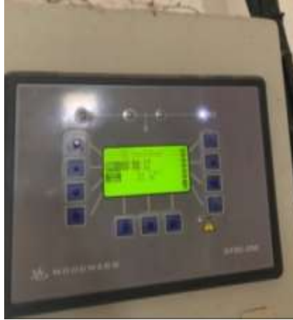
Gambar 2.5 Tampilan Modul WOODWARD DTSC-200
