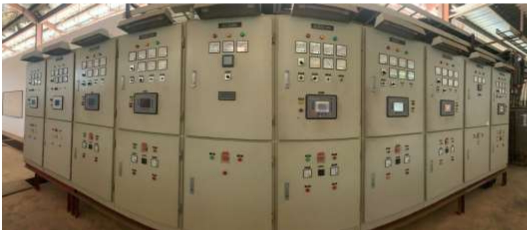
Gambar 3.6 Panel Sinkron
