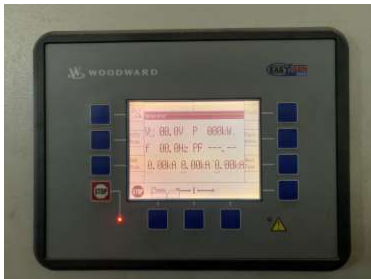
Gambar 3.8 Modul WOODWARD EASYGEN 3000
