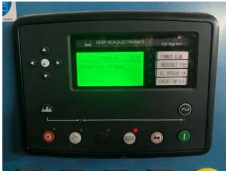
Gambar 3.7 Modul DEEP SEA ELECTRONICS DSE 8610 MKII
