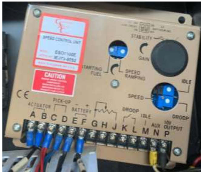
Gambar 3.9 AVR Speed Control
