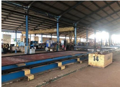
Gambar 1.9 Main Workshop Fabrication
