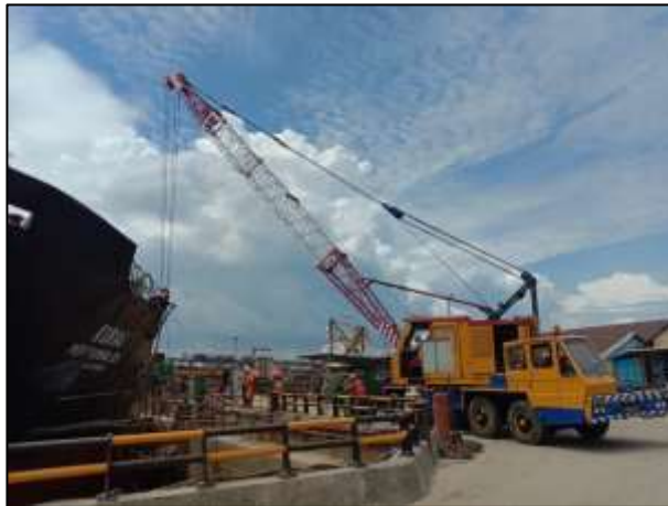
Gambar 1.8 Crawler crane PT. Yasa Wahana Tirta Samudera
