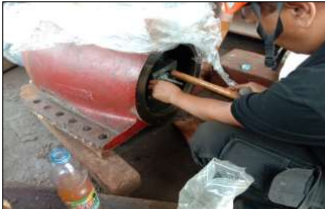
Gambar 2.135 Proses pemasangan Oil Distributor Box
