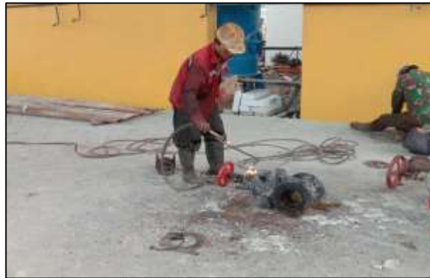
Gambar 2.88 Proses perbaikan ( repair ) valve
