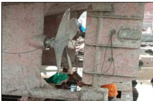
Gambar 2.46 Proses repair propeller kapal Sumber Marine 2
