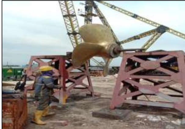
Gambar 2.33 Proses balansir propeller kapal TB. Patra Tunda 4201
