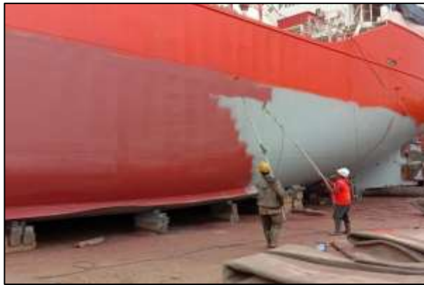
Gambar 2.57 Proses pengecatan Anti Fouling
