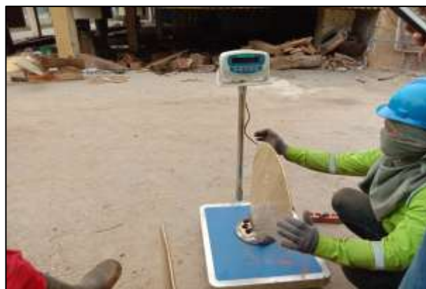
Gambar 2.133 Proses penimbangan daun propeller bow thruster
