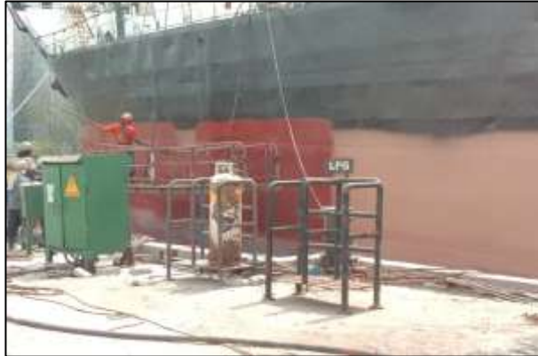
Gambar 2.53 Proses pengecatan Anti Fouling
