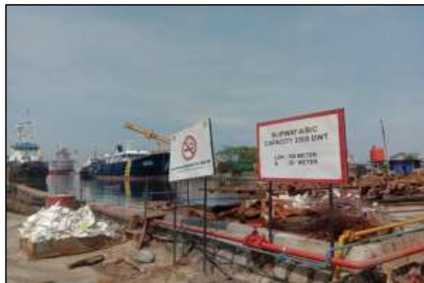
Gambar 1.12 Slipway A, B, C PT. Yasa Wahana Tirta Samudera
