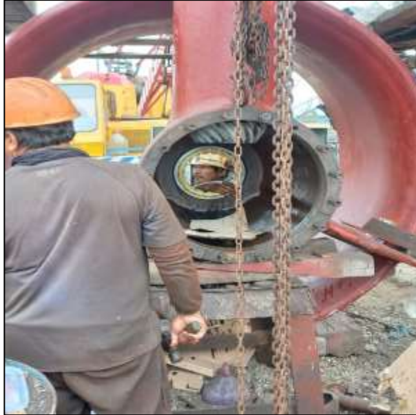
Gambar 2.35 Proses pemasangan bearing shaft propeller
