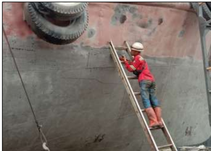
Gambar 3.2 Proses pengujian Ultrasonic Thickness Test
