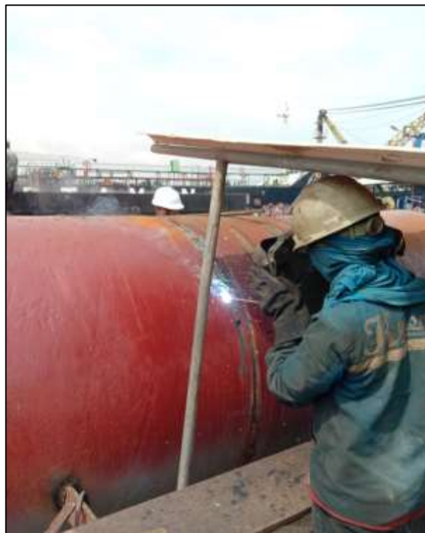
Gambar 2.26 Proses repair Stern Roller kapal Peteka 5402
