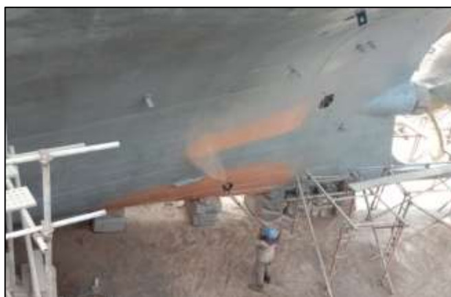
Gambar 2.152 Proses pengecatan tahap sealer/intermediate
