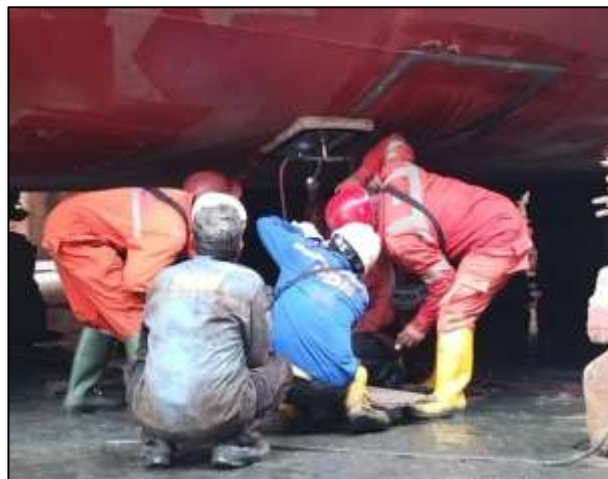
Gambar 2.42 Proses pengujian Vacuum Test
