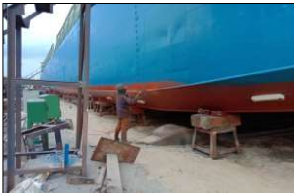
Gambar 2.124 Proses pengecatan anti fouling
