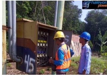
Gambar 2.31 Penimbangan Trafo (Sumber: PT. Haleyora Power, 2022)
