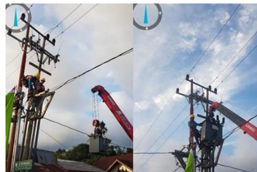
Gambar 2.42. Pengantian Trafo Gardu (Sumber: PT. Haleyora Power, 2022)
