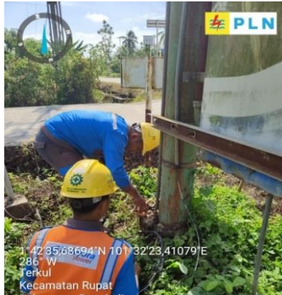
Gambar 2.3. Pemasangan Grounding (Sumber: PT. Haleyora Power, 2022)
