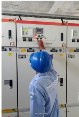
Gambar 2.12. Periksa Di GH (Sumber: PT. Haleyora Power, 2022)
