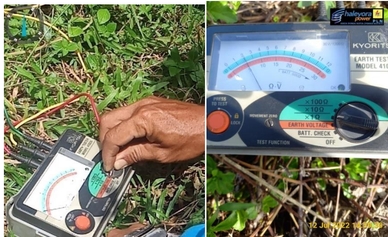
Gambar 2.16. Mengukur Tegangan Grounding (Sumber: PT. Haleyora Power, 2022)
