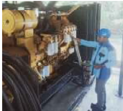
Gambar 2.21 Monitoring KWH (Sumber: PT. Megapower Makmur Tbk. 2022)
