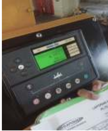
Gambar 2.18 Monitoring KWH (Sumber: PT. Megapower Makmur Tbk. 2022)
