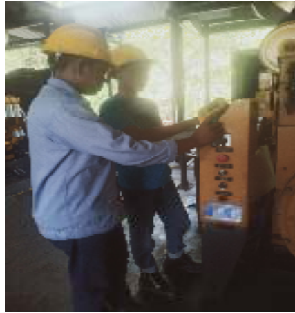
Gambar 2.6 Monitoring KWH (Sumber: PT. Megapower Makmur Tbk. 2022)
