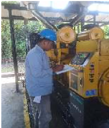
Gambar 2.15 Monitoring KWH (Sumber: PT. Megapower Makmur Tbk. 2022)
