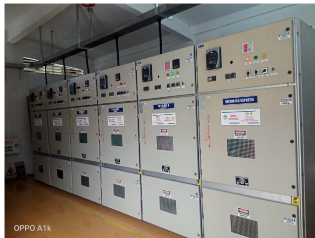
Gambar 2.29 Evident Beban Feeder
