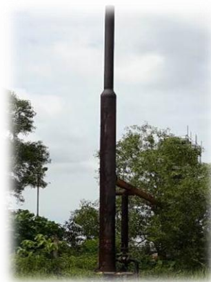
Gambar 3. 5 Test Vent Stack (Sumber: Power Point, 2022)
