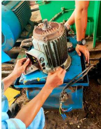
Gambar 2. 7 photo Open Install Motor 3 Phasa ( Suber: Dokumentasi 2022 )
