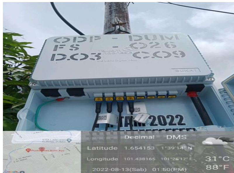
Gambar 3.2 Optical Distribution Point Sumber :(Dokumentasi,2022)
