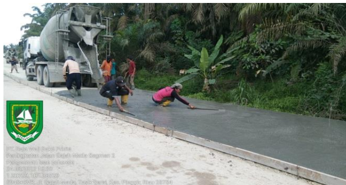
Gambar 3. 18 Pengecoran Lean concrete
