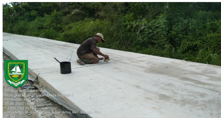
Gambar 3. 35 Pemberian joint sealant
