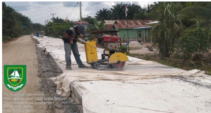
Gambar 3. 33 Cutting beton rigid
