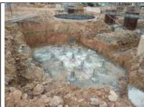
Gambar 3. 24 Proses Marking PC13
