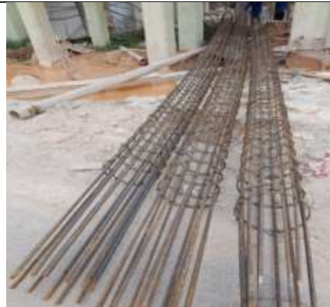
Gambar 3. 2 Spiral & rebar for borpile
