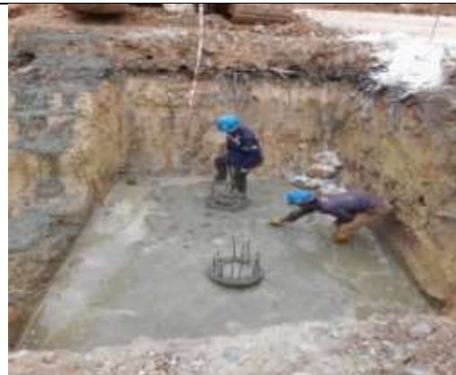
Gambar 3. 16 Pouring concrete k-100 to Lc piperack
