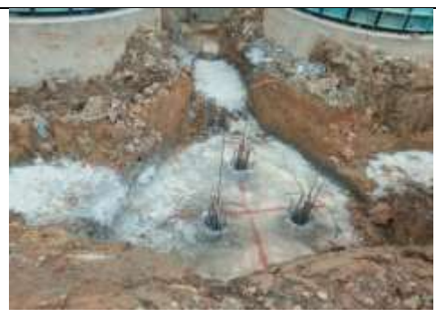
Gambar 3. 25 Proses marking pC3
