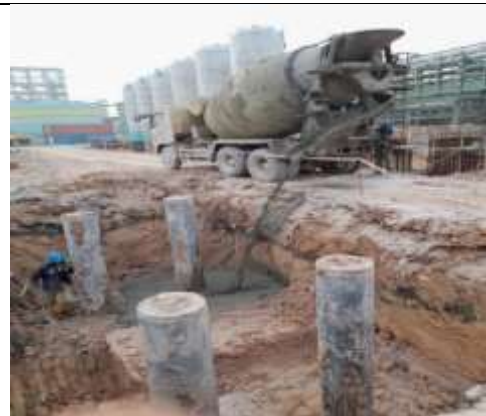
Gambar 3. 17 proses lean concrete k-100
