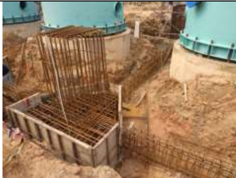
Gambar 3. 30 Proses Formwork Pc3
