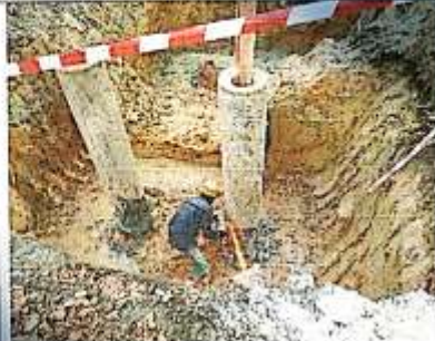
Proses cutting pile sebelum instal PHT.
