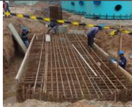
Gambar 3. 31 Proses Formwork Pc13
