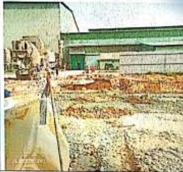
Penuangan lean concrete k-300
