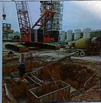
pouring concrete pile cape pipe rack
