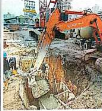
Pouring concrete k300 Piperack pilecape
