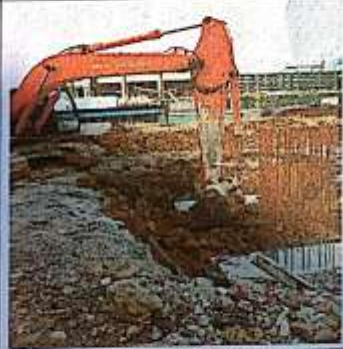
Proses pouring concrete k300 pedestal piperack dan penimbunan pilecapeee
