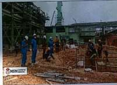
Proses cutting pile sebelum instal PHT.
