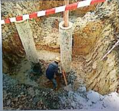
Proses cutting pile sebelum instal PHT.
