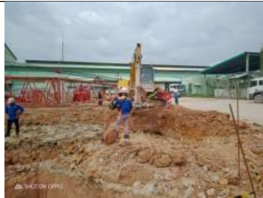
Gambar 3. 3 Penggalian building grid B
