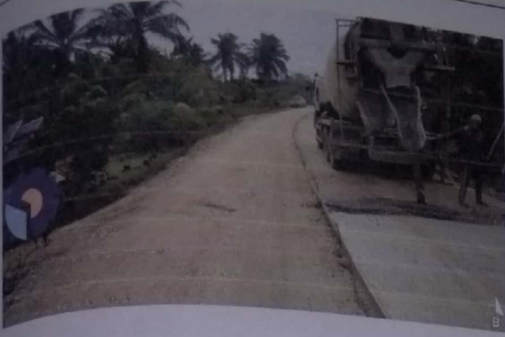
Pengecoran Lane Concrete STA 0+700 0+800
