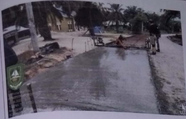
Pekerjan Rigid Pavement STA 1+100 - 1+200
