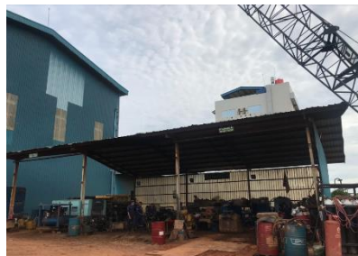
Gambar 1.10 Workshop Mechanical & Electrical
