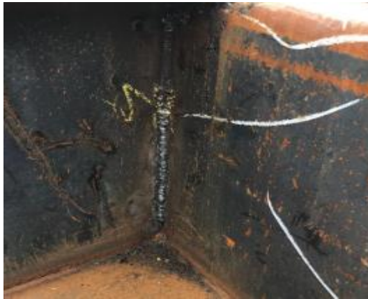
Gambar 2.105 Hasil visual welding inspect
