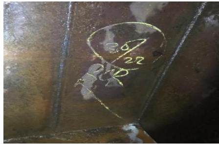
Gambar 2.45 proses air test
