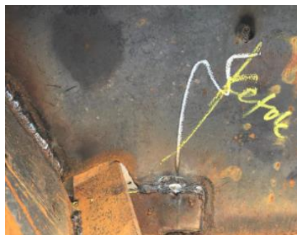
Gambar 2.66 Hasil visual welding inspect
