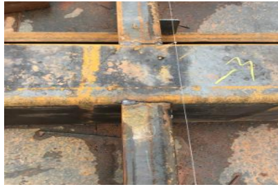
Gambar 2.103 hasil Fit Up check
