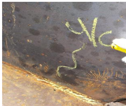
Gambar 2.95 visual welding inspect
