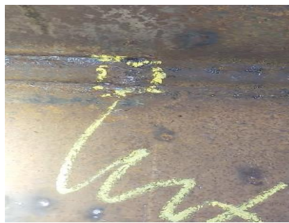
Gambar 2.49 Hasil visual welding inspect
