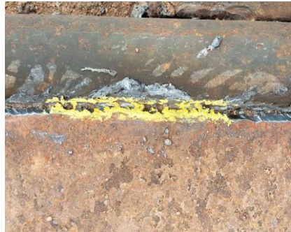
Gambar 2.83 hasil Visual welding inspect
