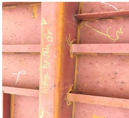
Gambar 2.54 Hasil Visual Welding Inspect
