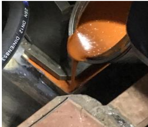
Gambar 2.71 penuangan cairan chockfast
