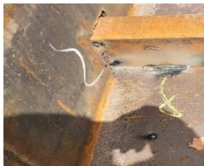
Gambar 2.51 hasil visual welding inspect
