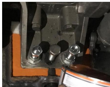
Gambar 2.44 penuangan orange chockfast
