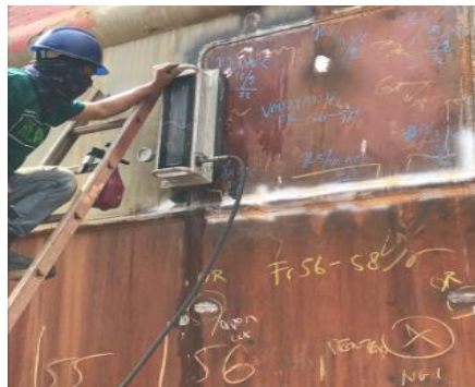
Gambar 2.18 Proses vacuum test
