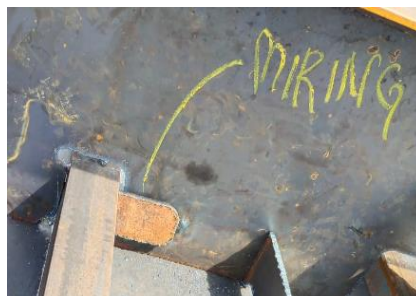
Gambar 2.33 hasil Visual Welding Inspect
