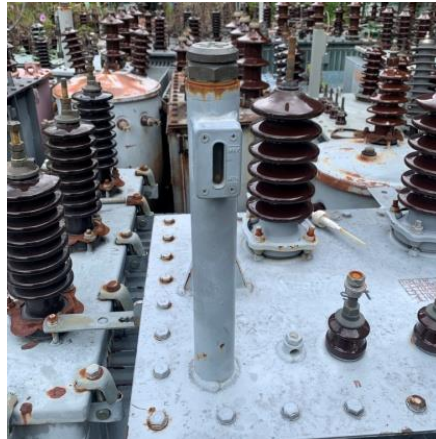
Gambar 3.4 Oil level Indicator (Sumber : PLN. Rayon Bengkalis PT. Adra gemilang. 2022)
