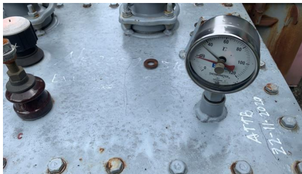
Gambar 3.5 Temperature Indicator (Sumber : PLN. Rayon Bengkalis PT. Adra gemilang. 2022)
