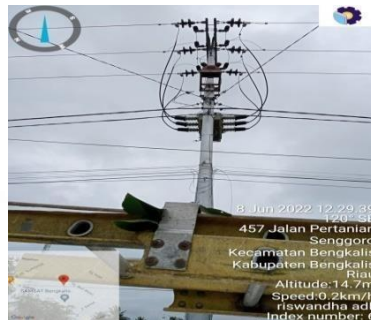
Gambar 2.6 Pengecekan LBS (load break switch )
