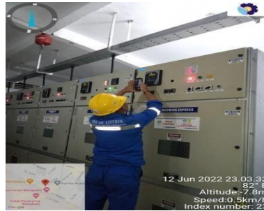
Gambar 2.8 Memfoto beban feeder
