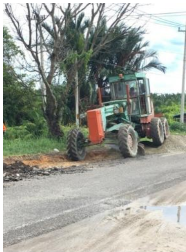
Gambar 3.5 Alat Motor grader
