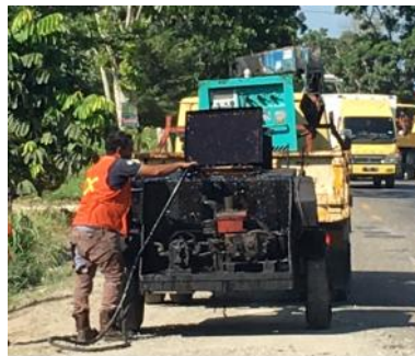
Gambar 3.9 Alat Asphalt sprayer
