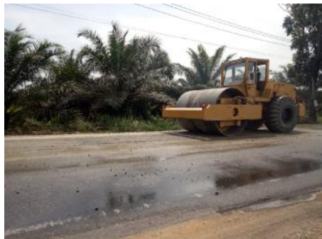
Gambar 3.3 Alat vibrator roller
