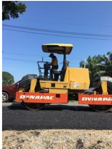
Gambar 3.11 Alat Tandem roller
