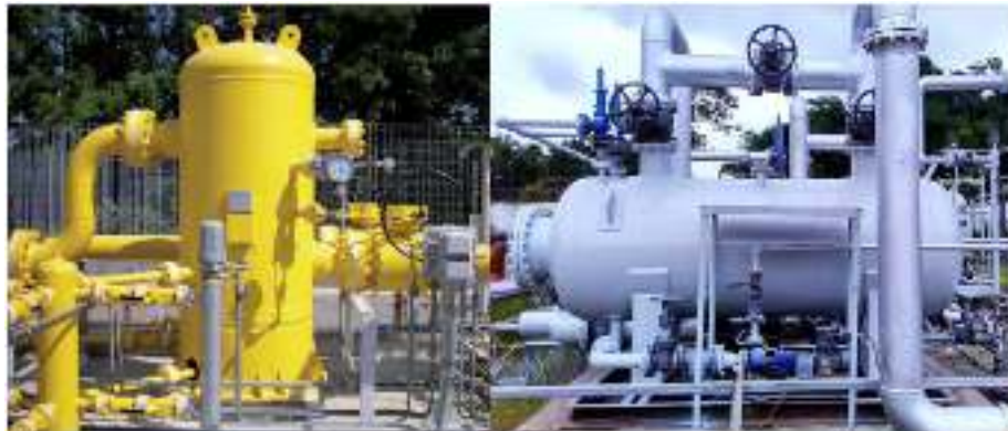
Gambar 3.1 KO Drum Vertical dan Horizontal (Sumber: https://amarineblog.com/2020/11/25/what-is-knockout-drum/ , 2022)
