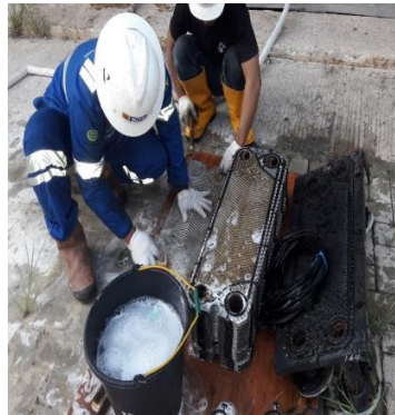
Gambar 4. 9 Cleaning plate Heat Exchanger
