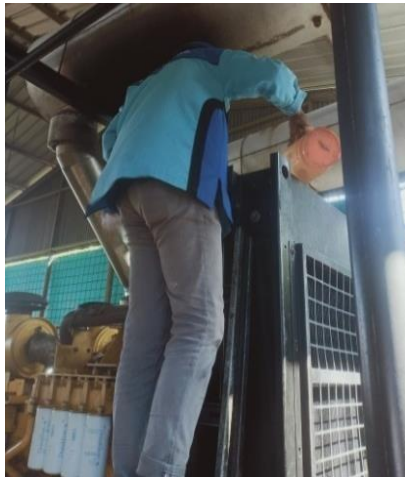
Gambar 2.21 Kegiatan penambahan air radiator (Sumber: PT. Megapower Makmur Tbk, 2022)
