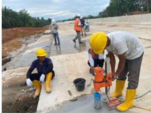
Gambar 3.14 Pengujian Core Drill
