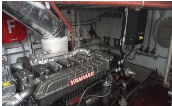
Gambar 2.20 Mengukur Main Engine
