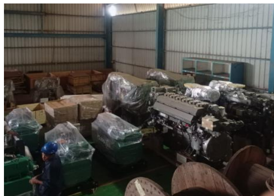
Gambar 2.24 Mengukur Main Engine Generator
