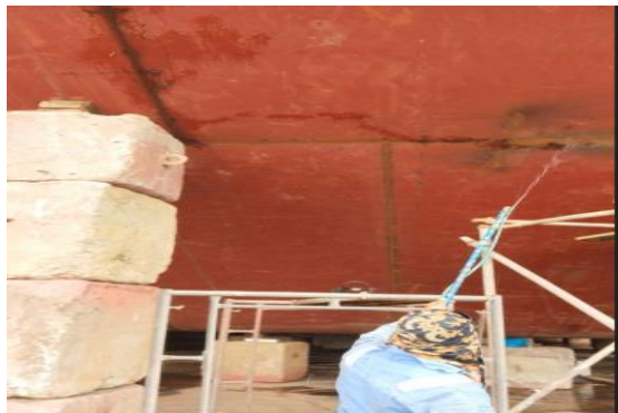
Gambar 2.69 Air Test External di Area Transom,Roun Bar dan Chain Plate
