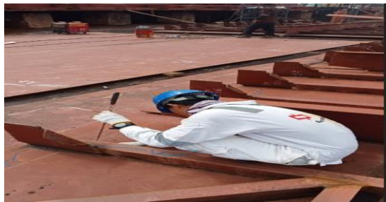
Gambar 2.59 Inspection Di Area Buttom Kapal Barge
