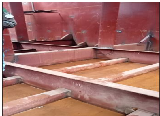
Gambar 2.62 Inspection Area Tangki Kapal Barge
