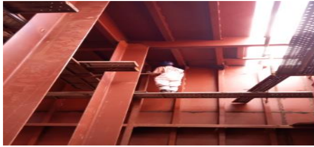
Gambar 2.70 Inspection Di Area Tangki
