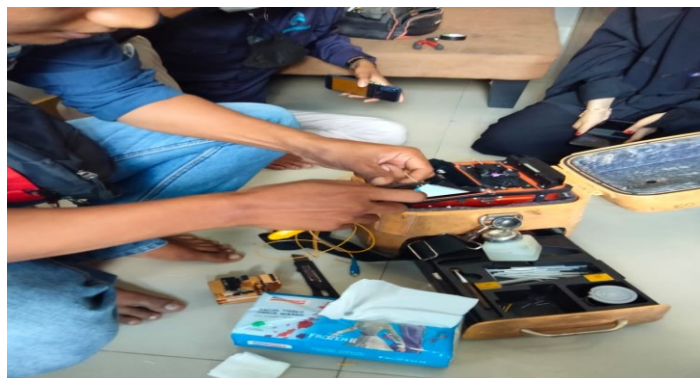
Gambar 3. 2 Metode Fusion Splice
