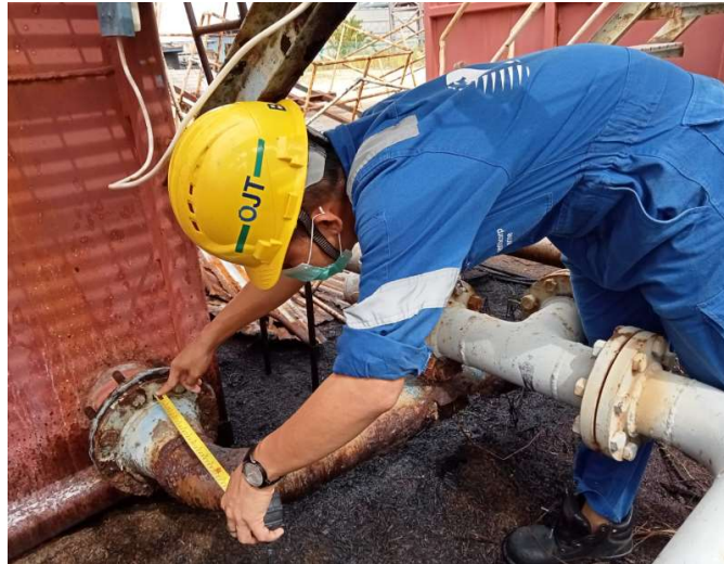
Gambar 2.36 Proses pengukuran pipa PT.KSS
