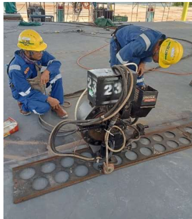
Gambar 3.8. Pengelasan SAW
