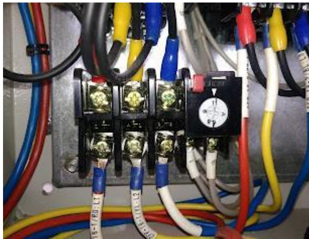
Gambar 3. 6 Thermal Overload Relay
