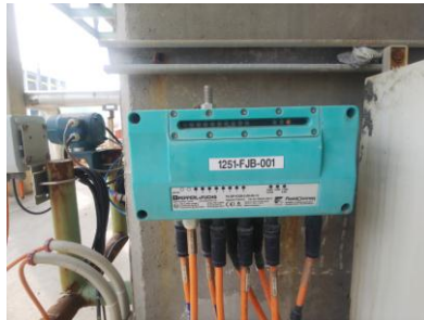
Gambar 2. 29 field bus junction box (FJB)
