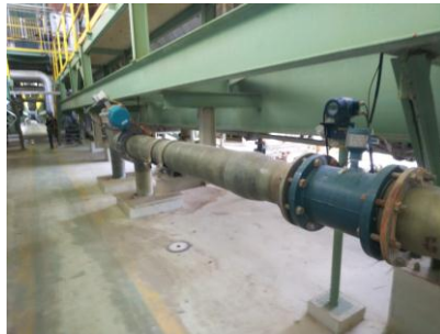
Gambar 2. 22 flow control evaporator
