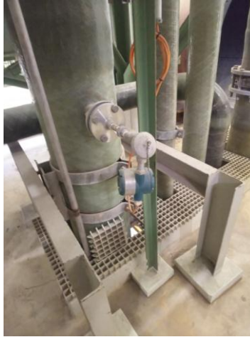
Gambar 2. 16 Temperature Transmitter evaporator
