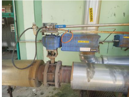
Gambar 2. 26 flow control valve
