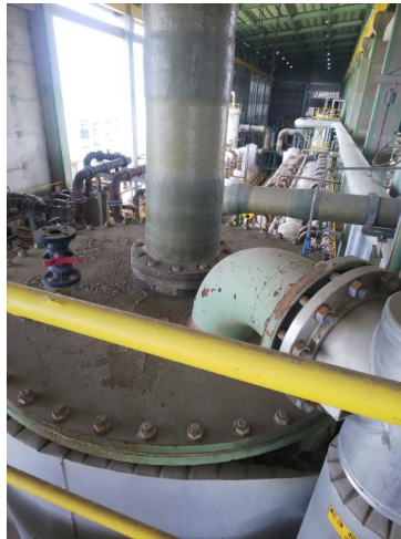
Gambar 2. 15 evaporator 3 spinbath
