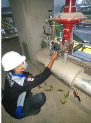
Gambar 2. 4 kalibrasi control valve
