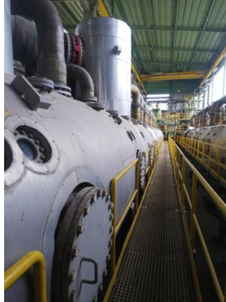
Gambar 2. 8 evaporator 3 spinbath
