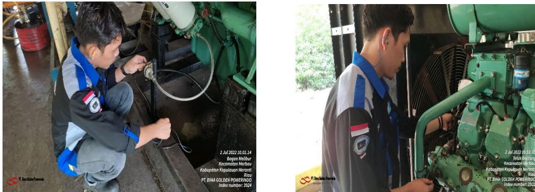
Gamabr 2.7 safety Device sensor water temperature dan sensor oil pressure
