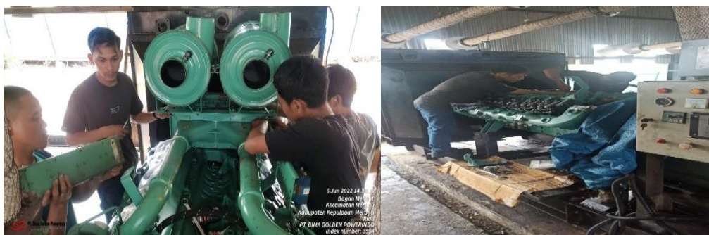
Gmbar2.4 Membantu GOH engine E#3
