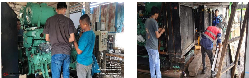
Gambar 2.2 Pengecekan engine dan pengecekan air radiator
