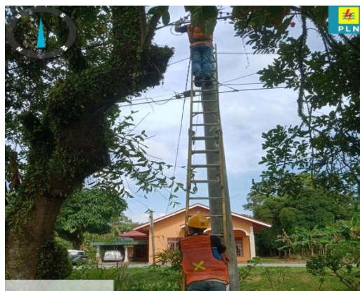
Gambar 2.22 Mengatasi Gangguan lost contact Nol/Netral
