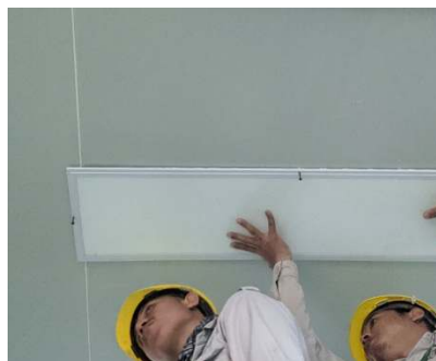
Gambar 2.11 Memasang LED Panel
