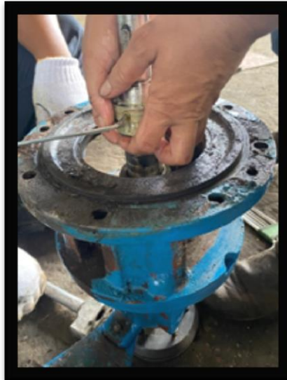
Gambar 4.13 Proses Pemasangan Mechanical Seal
