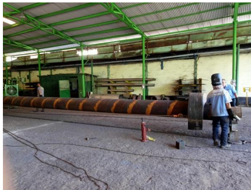
Gambar 4. 18 Proses Pemasangan Daun Screw Conveyor
