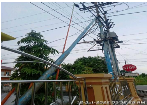
Gambar 2.17 Penggantian FCO ( Fuse Cut Out ) (Sumber: PT. Adra Gemilang 2022)
