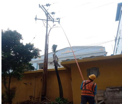
Gambar 2.5 Penggantian FCO ( Fuse Cut Out ) (Sumber: PT. Adra Gemilang 2022)
