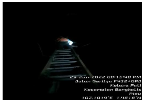
Gambar 2.12 Mengatasi Gangguan lost contact Nol/Netral (Sumber: PT. Adra Gemilang 2022)
