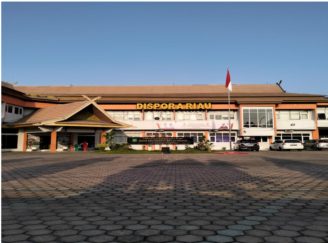
Figure 2.1 Building of Youth and Sports Department of Riau Province
