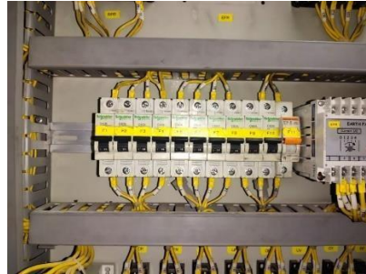
Gambar 3.3 MCB Kontrol Panel Sinkron (Sumber: PT. Megapower Makmur Tbk. 2021)
