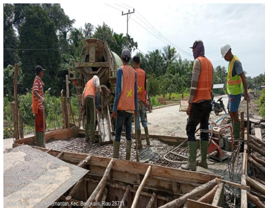
Gambar 3.8 pengecoran box culvert
