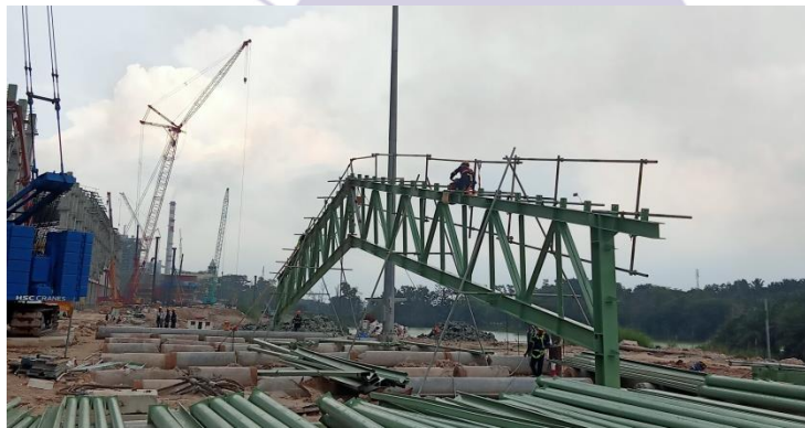
Gambar 3.46 penegakan rangka roofing truss
