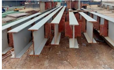
Gambar 3.21 beam gusset plate
