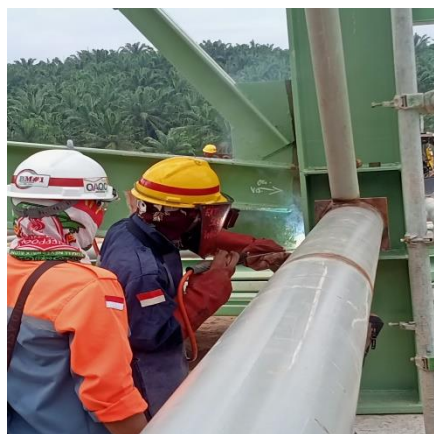
Gambar 3.51 welding finish truss
