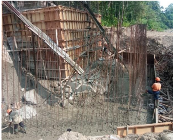
Gambar 3. 27 Pemasangan Retaining Wall Concrete
