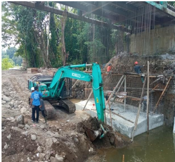
Gambar 3. 25 Galian Retaining Wall Concrete
