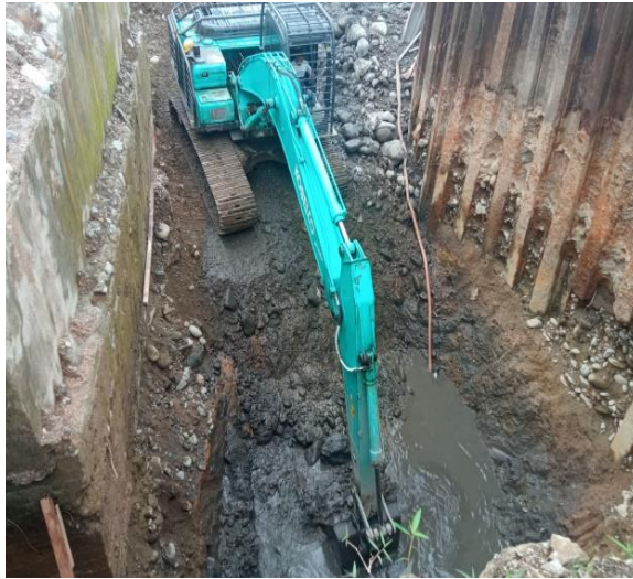
Gambar 3. 9 Galian Pondasi Sumuran
