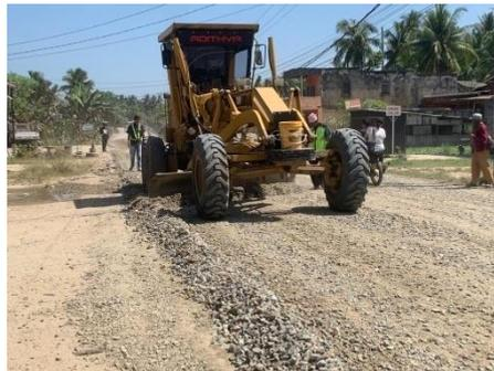
Gambar 3. 2 Motor Grader
