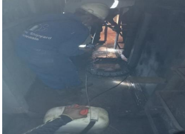
Gambar 2.22 Air Pressure Test
