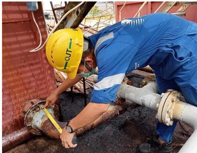
Gambar 2.35 Proses pengukuran pipa PT.KSS
