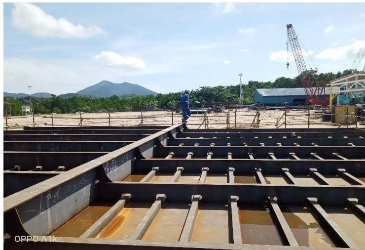
Gambar 2.46 pre-assembly panel -
