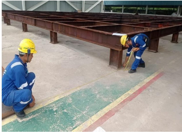
Gambar 2.19 Proses pengukuran layout PT.KSS
