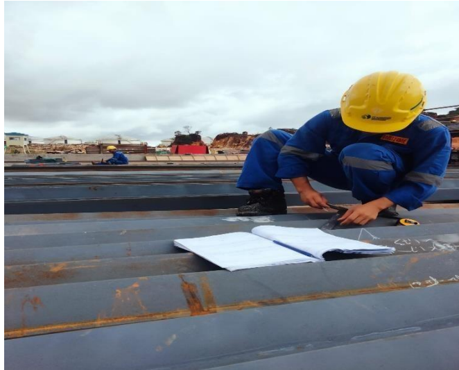
Gambar 2.45 Proses marking dilapangan
